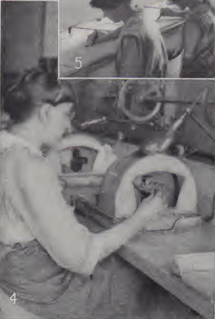
1—Gold melting and annealing furnaces. 2—Rolling gold to proper thickness before blanking for gold pen. 3—Showing strip of gold after blanking out gold pen. 4—Burring pen before tipping with iridium. 5—Grading and selecting iridium.
